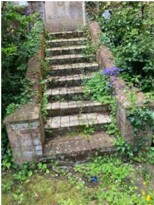
Photo 3 - Overgrown paths & stairways - dangerously uneven
